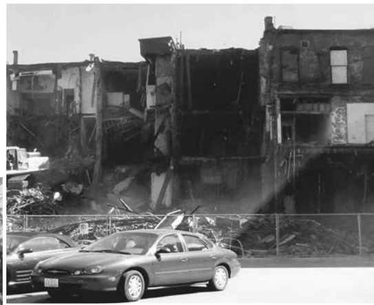
Demolition of buildings at 131 West Federal Street, between South Hazel and South Phelps streets, made way for construction of the Seventh District Court of Appeals.
