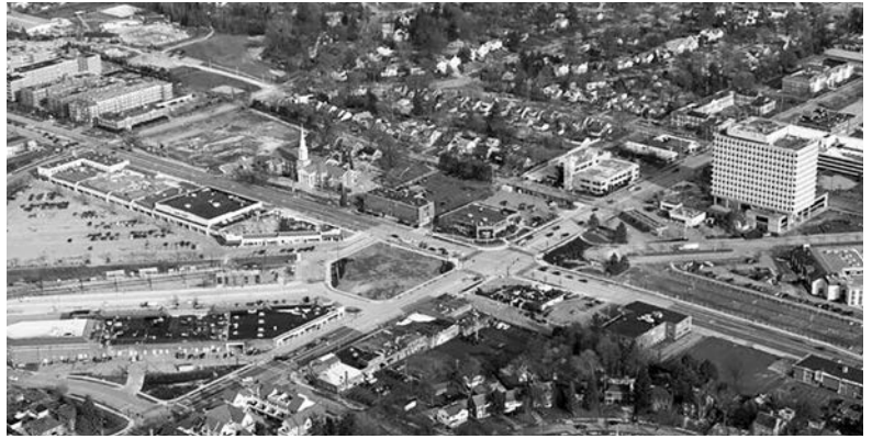
Aerial view of the Warrensville/Van Aken/Chagrin intersection largely complete in December 2015. The four way intersection with 90 second light timing is visible.
