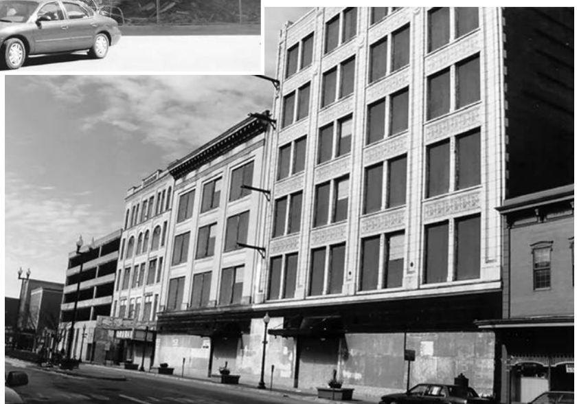
The parking garage for the long-vacant Higbee's department store building was in disrepair and had to be demolished due to its unstable condition. The Voinovich Government Center was erected in its place in 1999.
